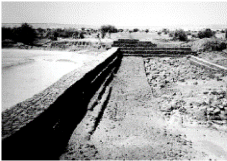
Fig. 2. A gabion weir
